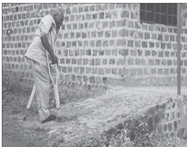
Figure 1. Concrete ramp providing access to classrooms
