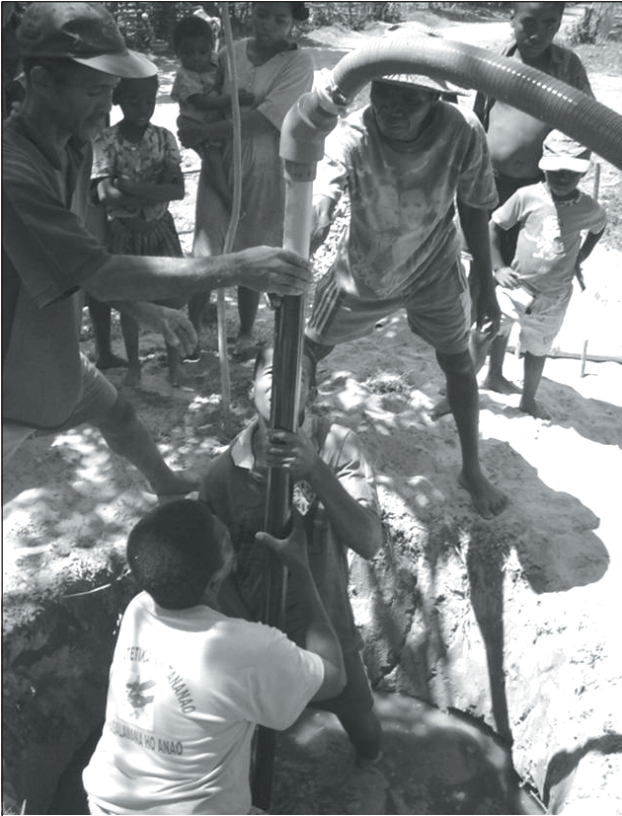
Photograph 1. It only takes about 2 minutes to jet a well screen 4 - 5 meters into the aquifer
