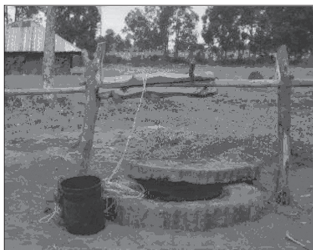
Figure 2. School water supply (before)
