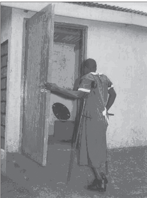
Figure 5. School latrine (after), showing concrete ramp, wide entrance and pedestal toilet
