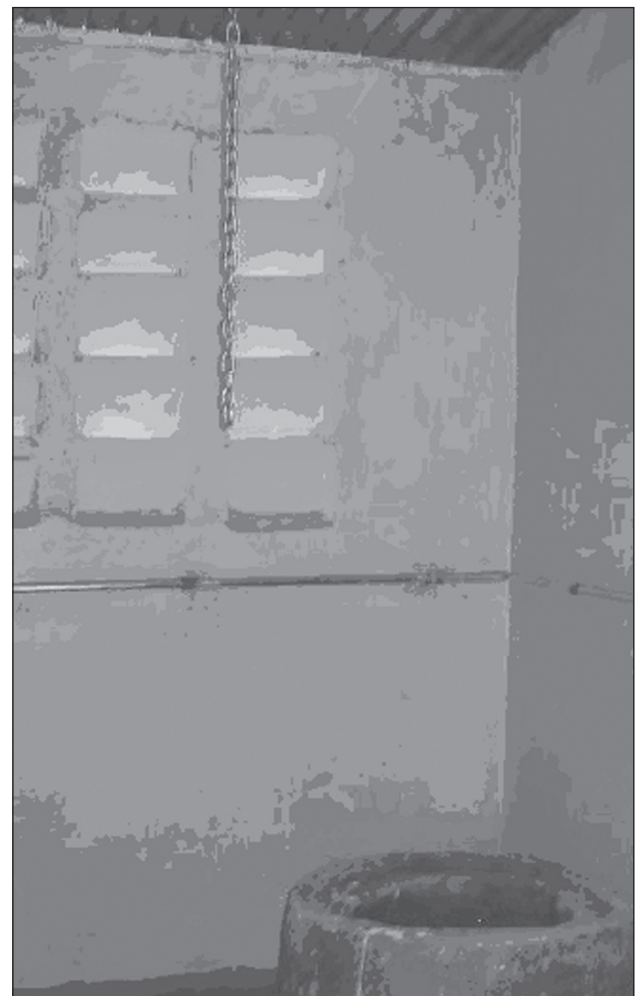
Figure 6. Interior of toilet showing handrails and chain from ceiling for support*
