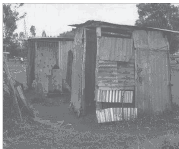
Figure 3. School latrines (before)
