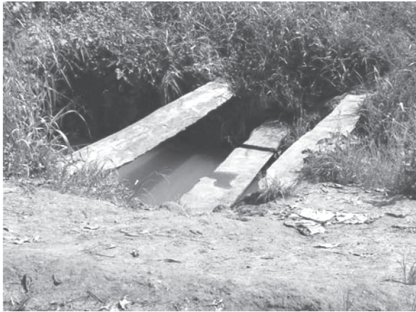
Photo 1. A “type 1” water source in Bugiri district
