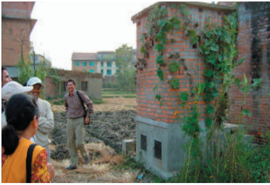
Photograph 3. ECOSAN toilet in use
