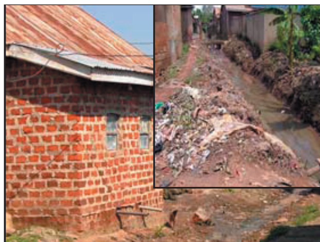
Figure 5. Figure 5: Sullage/storm water drain in the area with solid waste dumping on the drain bank (inset)
