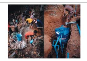
Photograph 2. Building of gabion intake with clay (left) and set up of plastic sedimentation tank (right)
