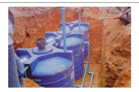
Photograph 3. Underground storage water tanks made from plastic (before earth filling)
