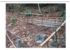
Photograph 1. Concrete intake and its overflow in Namhee Village (6 hrs walk from road access)
