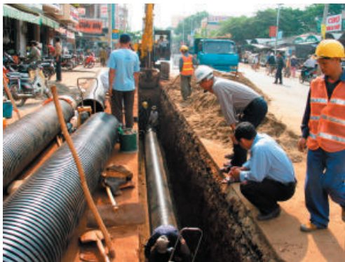
Figure 6. Installation of HDPE sewerage piping
