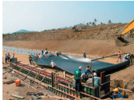
Figure 7. HDPE lining of stabilization pond
