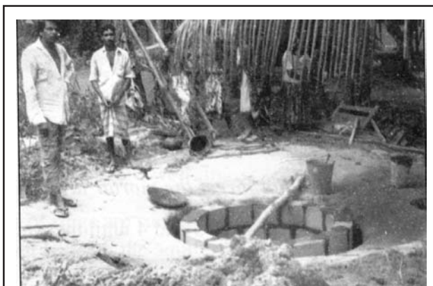
Figure 2. Dugwell lined with sandcrete blocks
