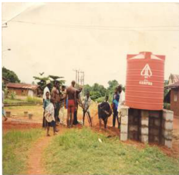
Picture 3: The balancing overhead storage tank – this helps in distributing the water by gravity
