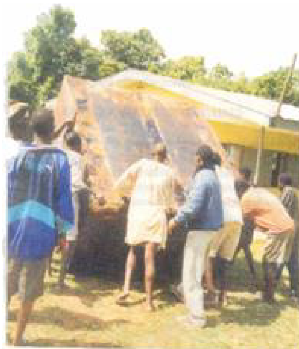
Picture 2. The 2000 gallons steel tank being taken away from its original platform
