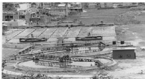
Figure 2. Oxidation ditch and secondary clarifier
