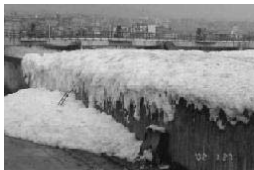
Figure 3. Foam in oxidation ditch
