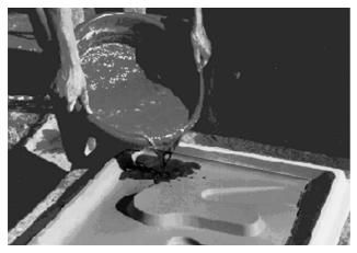
The small SanPlat 60x60 cm is easily made in an all-in-one plastic mould For best results the first portion of concrete should be a cement slurry later much stiffer concrete (1+2+2 volumes of cement sand and stone) is added to absorb the excess water
