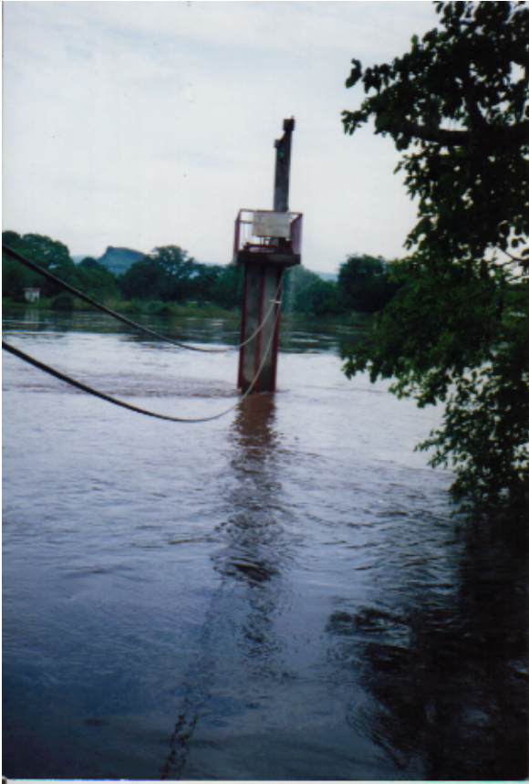
Figure 3. Infiltration gallery under operation
