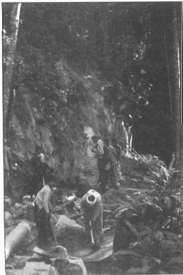
Photograph 1. Construction of a bench and concrete pipeline
