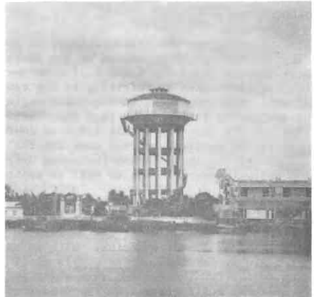
Pump house and overhead storage tank
