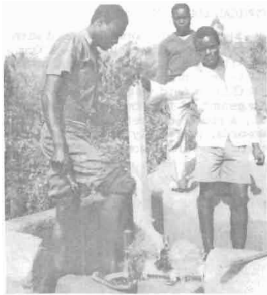
Spring protection furnished with a locally made hydram.
