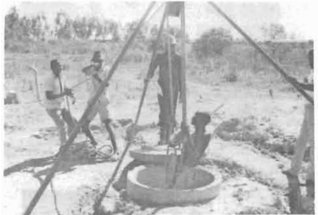
Hand-digging of a well
