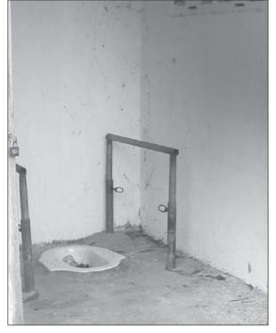
Figure 7.43. Squat toilet installed level with the surrounding floor. (Case-study 9.16, page 207)
