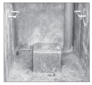
Figure 7.3. Handrails cemented to each side wall of toilet cubicle. H:  $\sim$  80cm – likely to be too high and too far apart for some child users. (Case-study 9.29, page 242)
