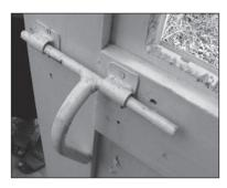
Figure 9.123. Large slide bolt for easy grip.
