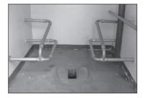
Figure 9.125. Squat latrine with handrails for support.
