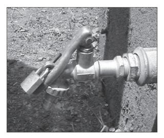
Figure 6.22. Lever operated tap with padlock. Unsuitable for a person with limited grip or stiff fingers.
