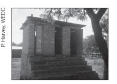
Figure 2.4. Latrine in Tanzania with steep steps and narrow doors.
