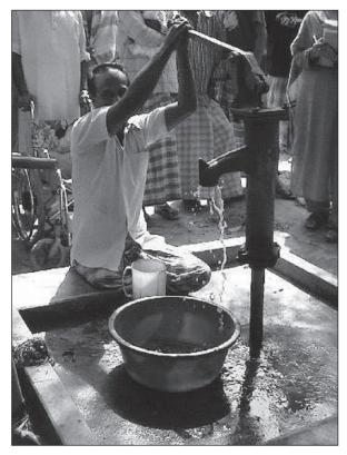
Figure 6.3. Low concrete sitting platform built into pump apron. *(Case-study 9.2, page 161)*
