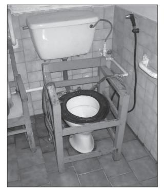
Figure 7.12. Painted wooden frame around pedestal toilet seat.
