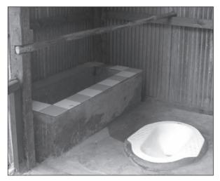
Figure 7.53. Water trough inside toilet cubicle. (Case-study 9.19, page 215)
