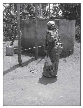
Figure 5.13. Two fixed wooden posts act as landmarks for a blind woman to find her way to and from the water tank or toilet. For a user with some vision, posts could be painted/marked a bright colour.
