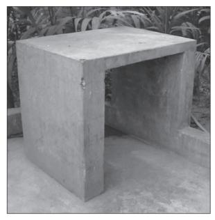
Figure 6.83. Concrete slab for washing clothes. (Case-study 9.3, page 166)
