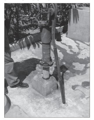
Figure 6.4. Handpump with apron showing direction of water drainage away from pump. Note lengthened handle for extra leverage. *(Case-study 9.3, page 164)*
