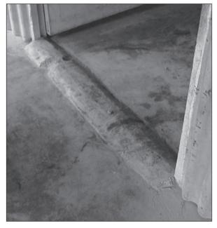
Figure 5.14. Low threshold for flood prevention, rounded for easy wheelchair access. *(Case-study 9.4, page 169)*
