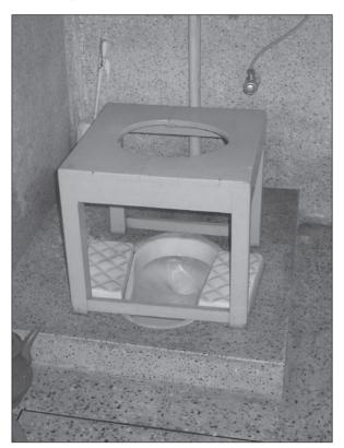
Figure 7.36. Toilet stool used over a squat toilet. Painted wood resists moisture. No splash-guard.
