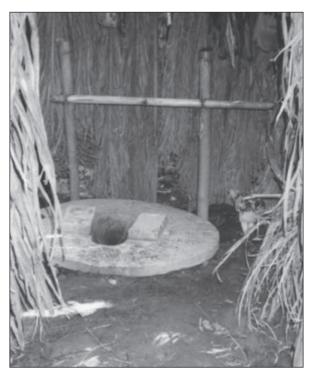
Figure 7.9. Single horizontal bamboo rail in front of toilet. (Case-study 9.10, page 185)
