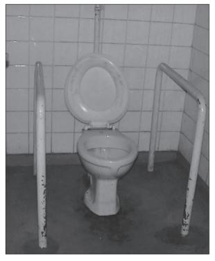
Figure 7.2. Painted handrails cemented to floor on both sides of pedestal toilet. 50mm  $\emptyset$  g.i. pipe; H: ~80cm.
