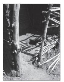
Figure 9.132. The packed earth floor of the pit latrine.
