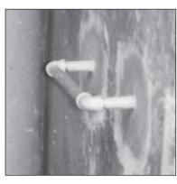
Figure 9.144. Handrail cemented to the wall.
