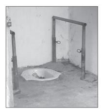
Figure 9.80. Adjustable handrails.
