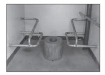
Figure 9.124. Raised toilet seat with handrails for support.
