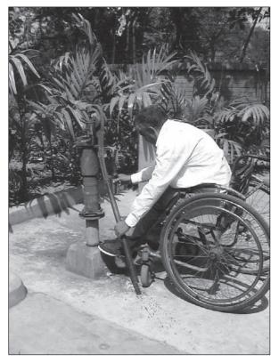
Figure 6.5. The same handpump operated by a wheelchair user on a level apron. *(Case-study 9.3, page164)*
