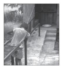
Figure 9.94. Horizontal parallel bars enable child to walk from house to toilet with minimal help
