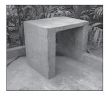
Figure 9.16. Concrete laundry slab located on edge of handpump apron.
