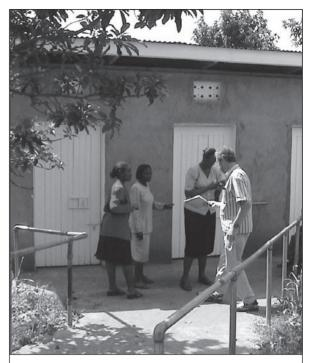
Figure 5.10. Wide concrete ramp with handrails both sides.
