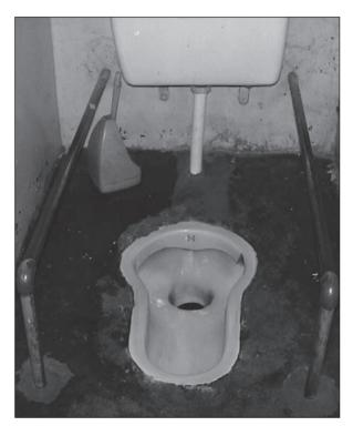
Figure 7.1. Handrail attached to floor on both sides of a squat toilet. H:  $\sim$ 30cm. (The wide toilet pan is not recommended.)
