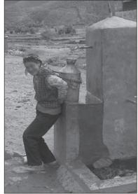
Figure 9.160. 'Back-happy' tapstand in use. Note direction of water drainage into groundlevel splash apron.
