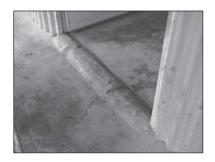
Figure 9.24. Flood prevention threshold has been rounded for easier wheelchair access.
