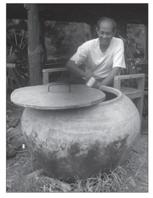
Figure 6.35. Ferrocement water storage jar. Water is scooped from the top using a mug. (Case-study 9.17, page 209)
