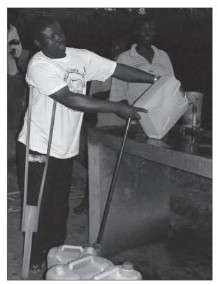
Figure 6.17. Taps  $\sim$ 25cm above a concrete shelf (H:  $\sim$ 1m) do not require the user to bend. (Case-study 9.20, page 217)
