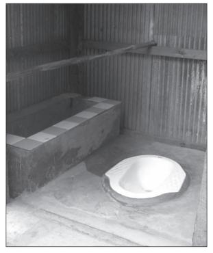
Figure 7.6. Single horizontal wooden rail (H:  $\sim$ 50cm) from door to back wall, for support to enter toilet. Too high for child to hold while squatting.
