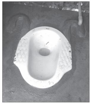
Figure 7.42. Cement mortar mouldings next to toilet pan for wheels of wheelchair to slot into for accurate positioning. *(Case-study 9.15, page 201)*
