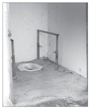
Figure 7.17. Handrails of adjustable height, suitable for a growing child. (*Case-study 9.16, page 207*)
