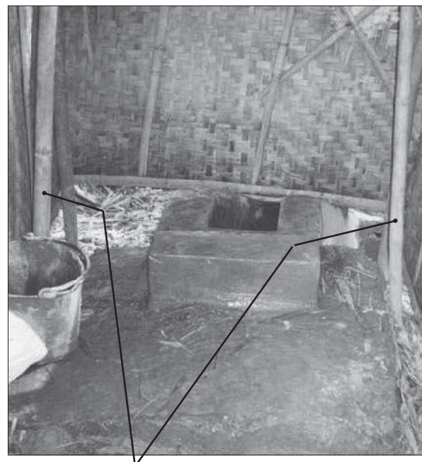
Figure 7.11. Two vertical bamboo support poles one on each side of latrine. (Case-study 9.9, page 183)
