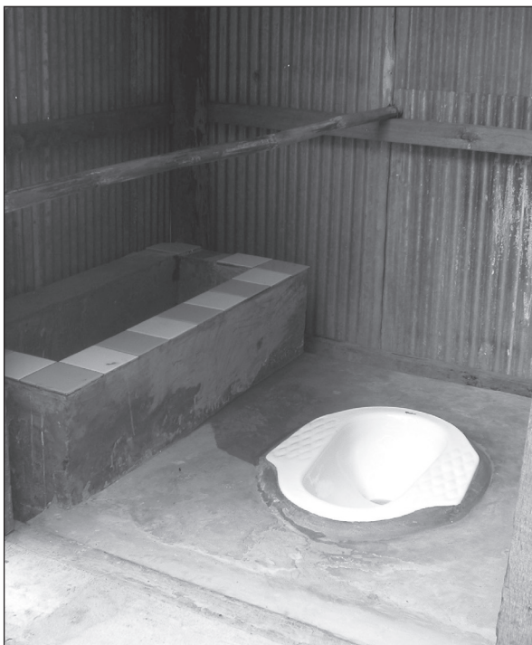
Figure 7.6. Single horizontal wooden rail (H: ~50cm) from door to back wall, for support to enter toilet. Too high for child to hold while squatting.
