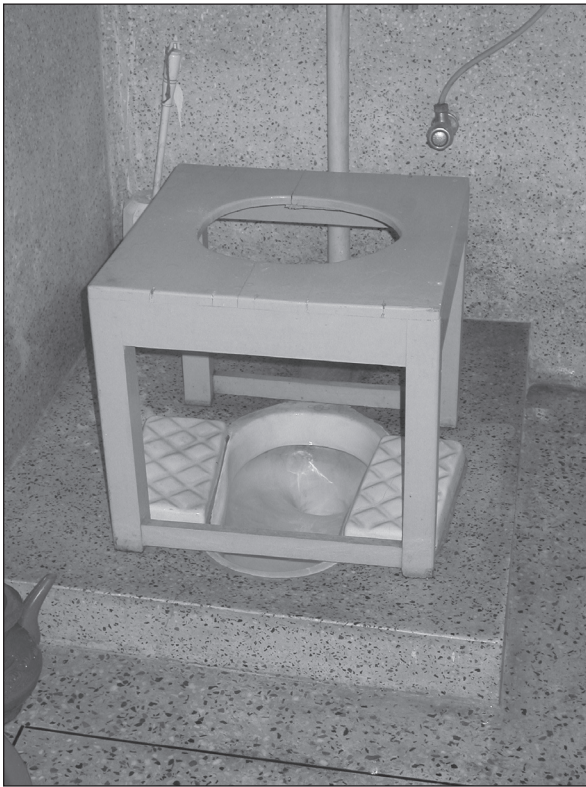
Figure 7.36. Toilet stool used over a squat toilet. Painted wood resists moisture. No splash-guard.
