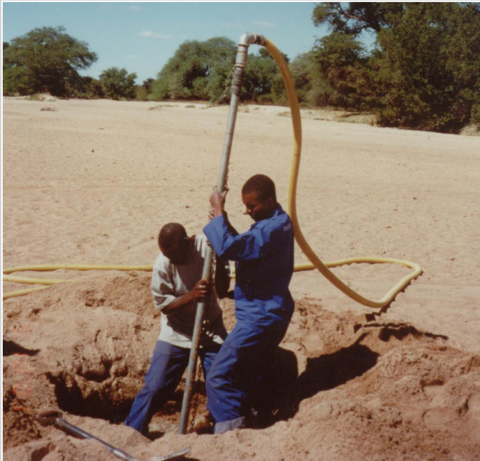
Photograph 5.8. Installing a self-jetting well-point
