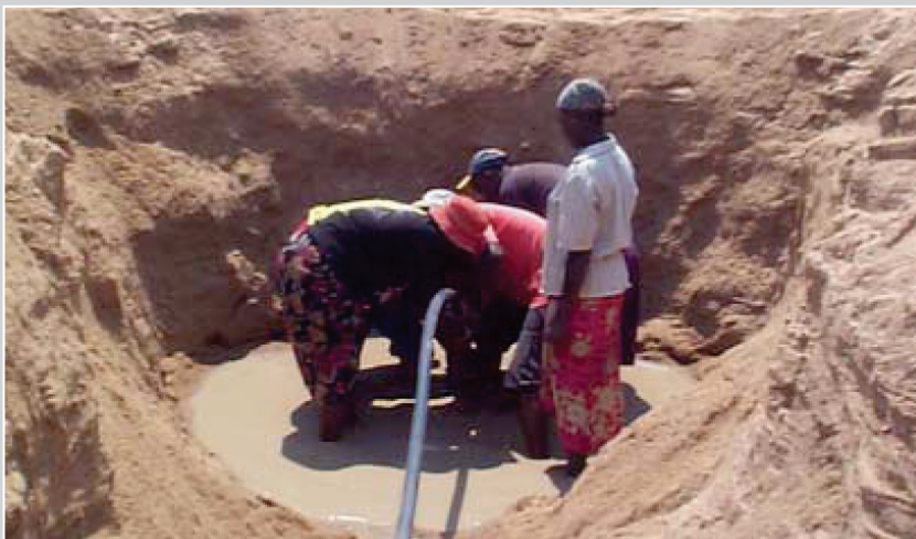
Photograph 5.5. Digging in a well-point
