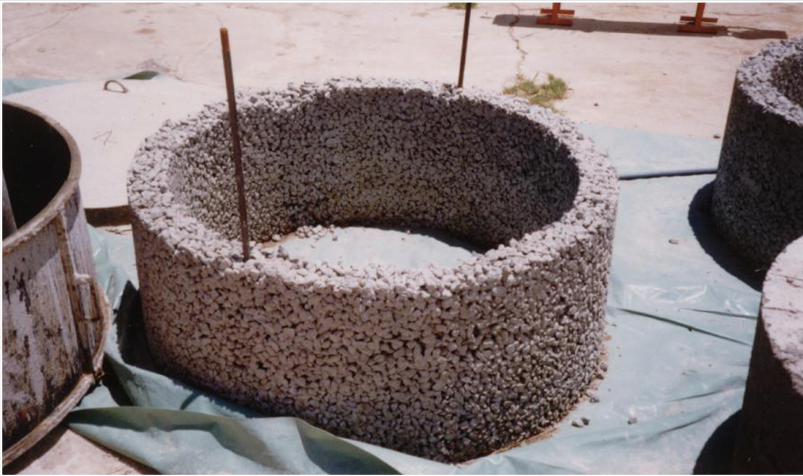
Photograph 5.3. No fines concrete well-screen
