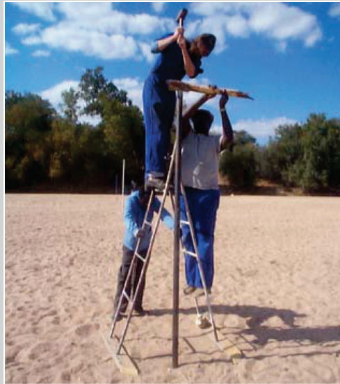
Photograph 5.6. Driving in a well-point to 3 metres
