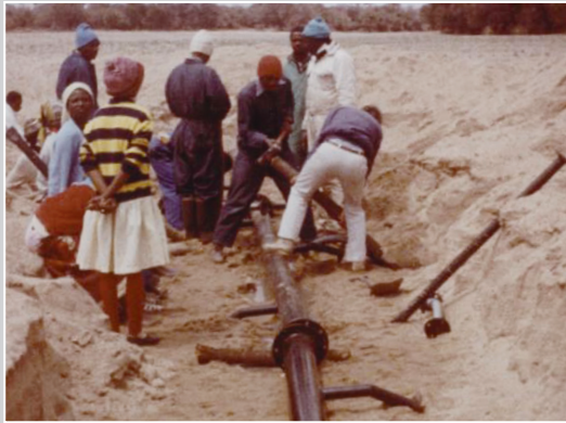
Photograph 5.4. Installation of a multiple well-point system
