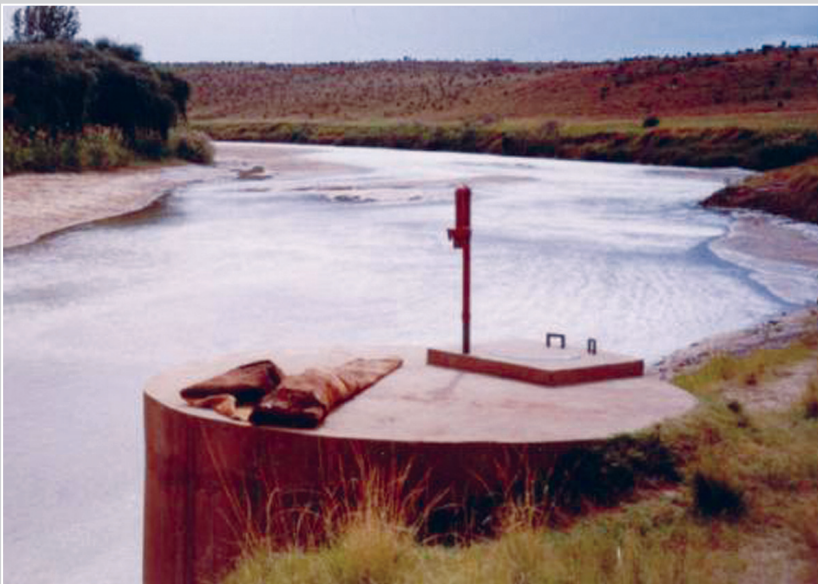
Photograph 5.7. Infiltration gallery and collector well on Blood River, South Africa
