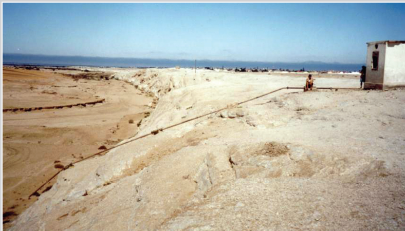
Photograph 4.11. Sub-surface dam Swakop River, Swakopmund, Namibia
