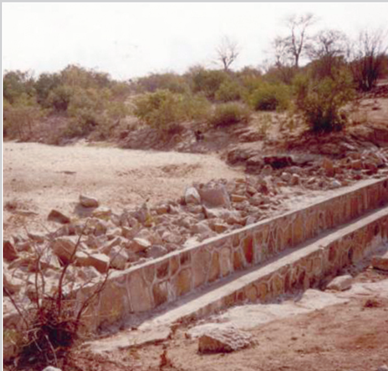
Photograph 4.10. Mkayi Wokhoza sand dam under construction
