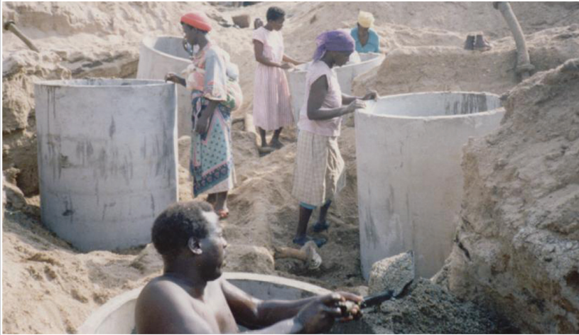
Photograph 4.9. Installation of concrete caissons in the Rundi River, Zimbabwe
