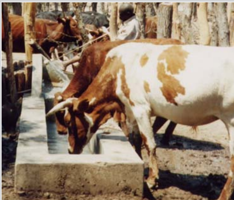
Photograph A1.2. Makhulela community sand-abstraction water supply
