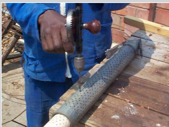
Photograph A1.1. Use of a jig in the construction of well-points
