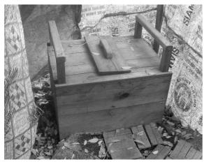
Figure 18. Wooden toilet seat installed over latrine pit (SCI Centre, Battambang).
