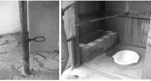
Figure 16. Adjustable handrail made of iron pipe (HI/CABDIC).
