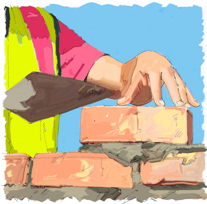
Figure 1. Laying cement and bricks
