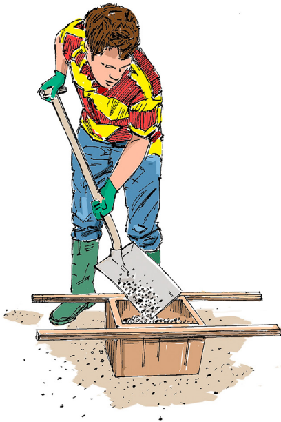
Step 2. Filling the container with aggregate
