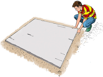
Step 1. Laying out the board
