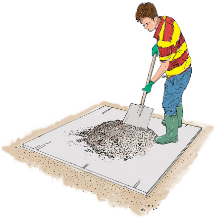
Step 6. Mixing the aggregates and cement together
