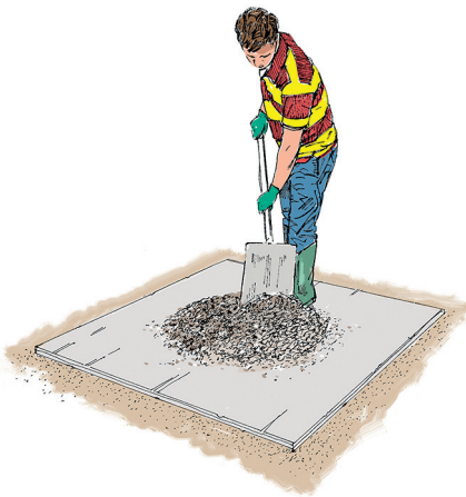
Step 9. Mixing the pile again
