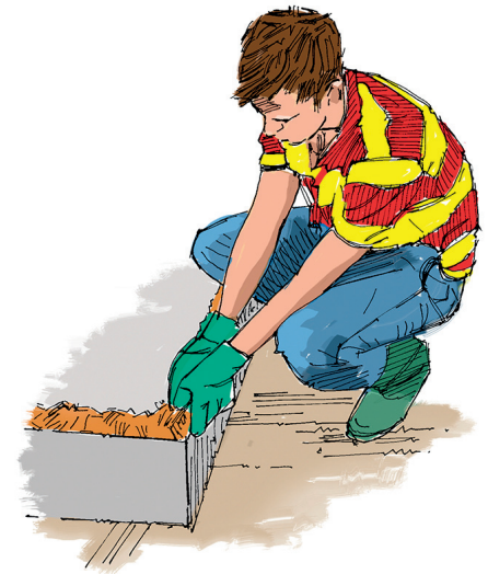
Figure 8. Constructing a clay dam
