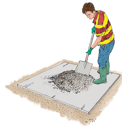
Step 6. Mixing the aggregates and cement together
