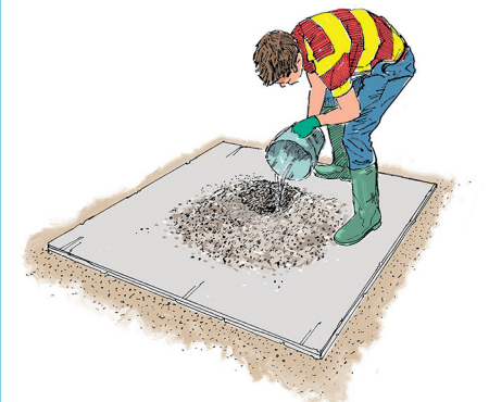
Step 8. Pouring water into the crater
