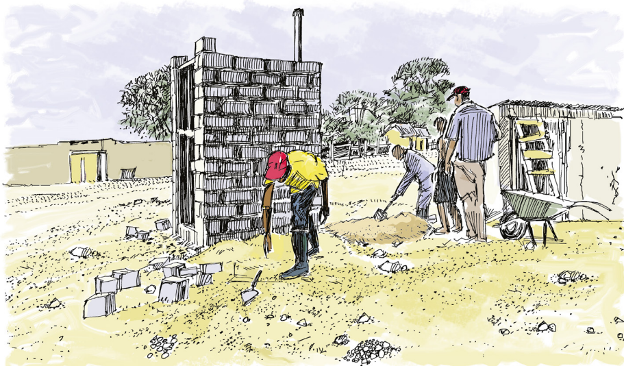
Figure 6. A VIP latrine under construction
