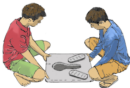
Figure 18. Lifting a sanplat
